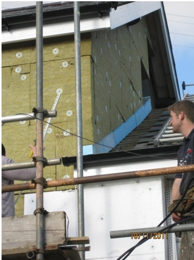
PU slab in splash zone (on roof)
