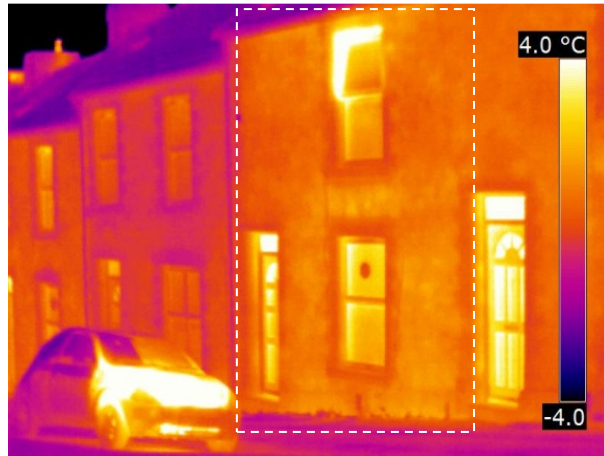
Figure 7: Pre-R:T survey image of dwelling, as shown in Figure 6
