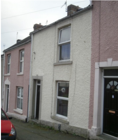
Figure 6: Photograph of dwelling before installation of insulation
