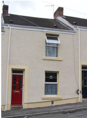
Figure 8: Photograph of dwelling shown in Figure 6, after installation of insulation
